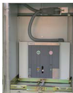
Circuit breaker compartments
