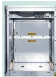
Circuit breaker compartment metal shutter
